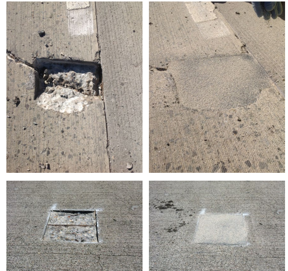
FastPatch 5000 Kit Compression Strength: ASTM C579 Method B, 2" cubes
